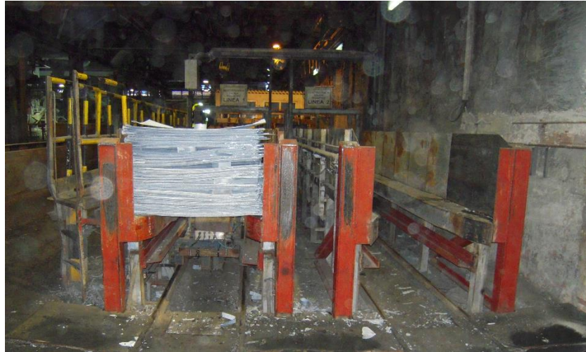
Picture 13. Bundle Outlet Conveyor
